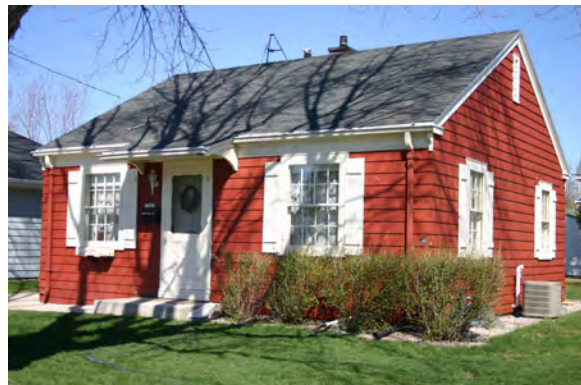
Side gable residence, 1302 Western Street
