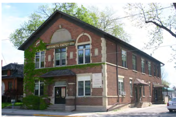
Romanesque Revival Sons of Herman Building, 316 Court Street (reevaluation property)
