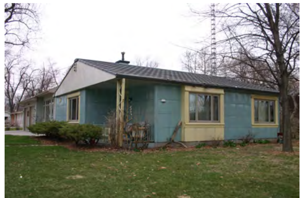
Lustron residence, 1020 Baldwin Avenue
