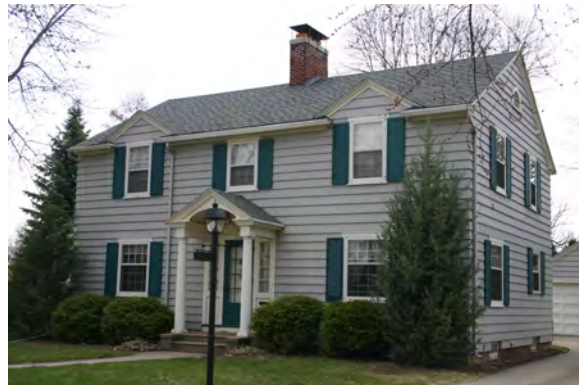
Colonial Revival residence, 1109 Bowen Street
